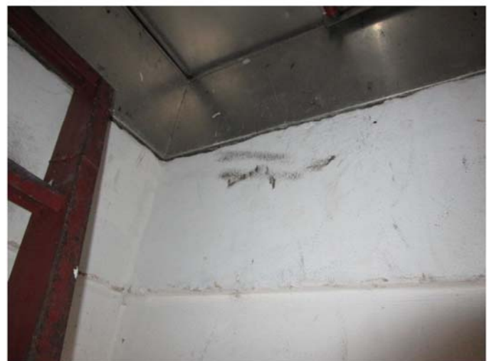
CONCRETE ROOF DECK
