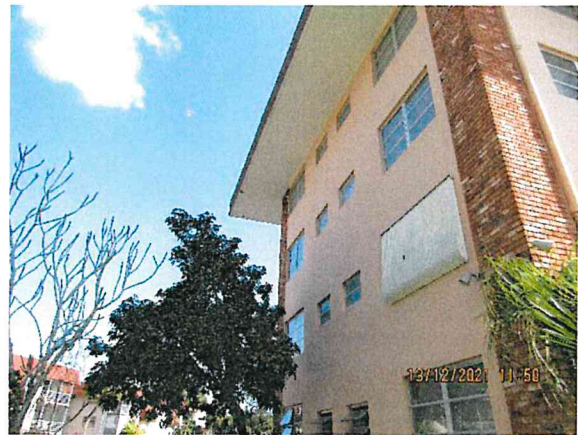
5: View of the north elevation of the subject building; facing east.
