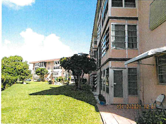
7: View of the west elevation of the subject building; facing north.
