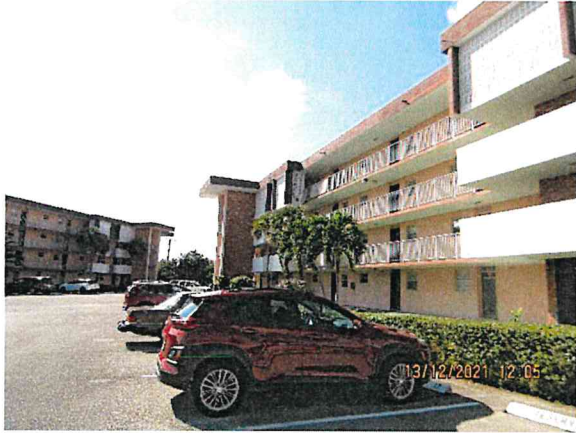
10: View of the southeast elevation of the subject building; facing southwest.
