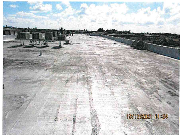
11: View of the roof of the subject building.
