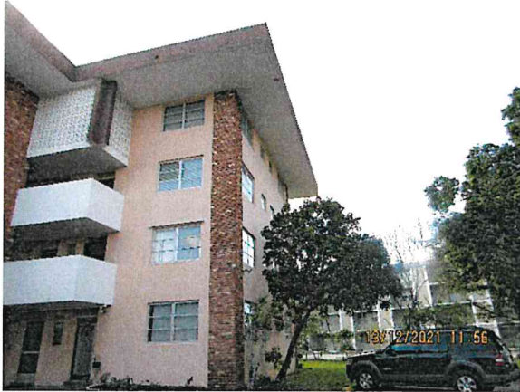
4: View of the north elevation of the subject building; facing west
