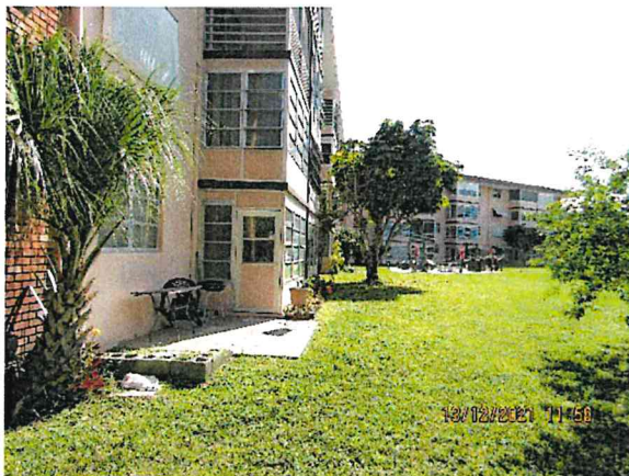
6: View of the west elevation of the subject building; facing south
