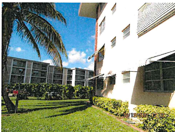
9: View of the south elevation of the subject building; facing west.
