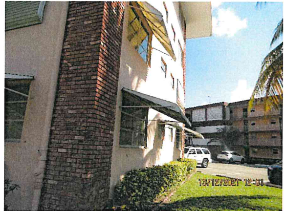
8: View of the south elevation of the subject building; facing southeast.
