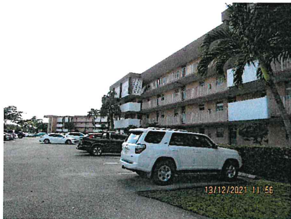
3: View of the northeast elevation of the subject building; facing south.
