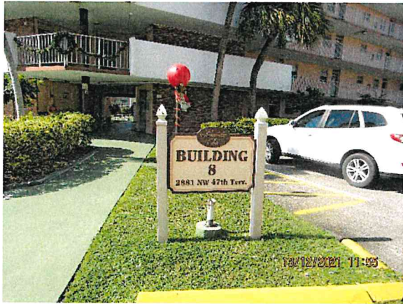
1: View of the east entrance to the subject building; facing west.
