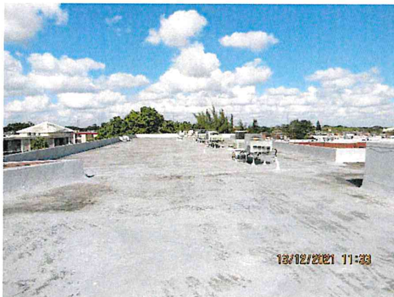
12: View of the roof of the subject building.
